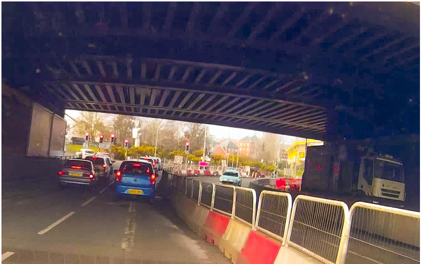
The roadworks at Colchester north station
